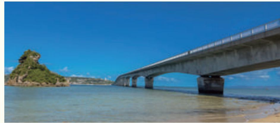
【今帰仁村】古宇利大橋 Nakijin Village / Kouri Bridge
